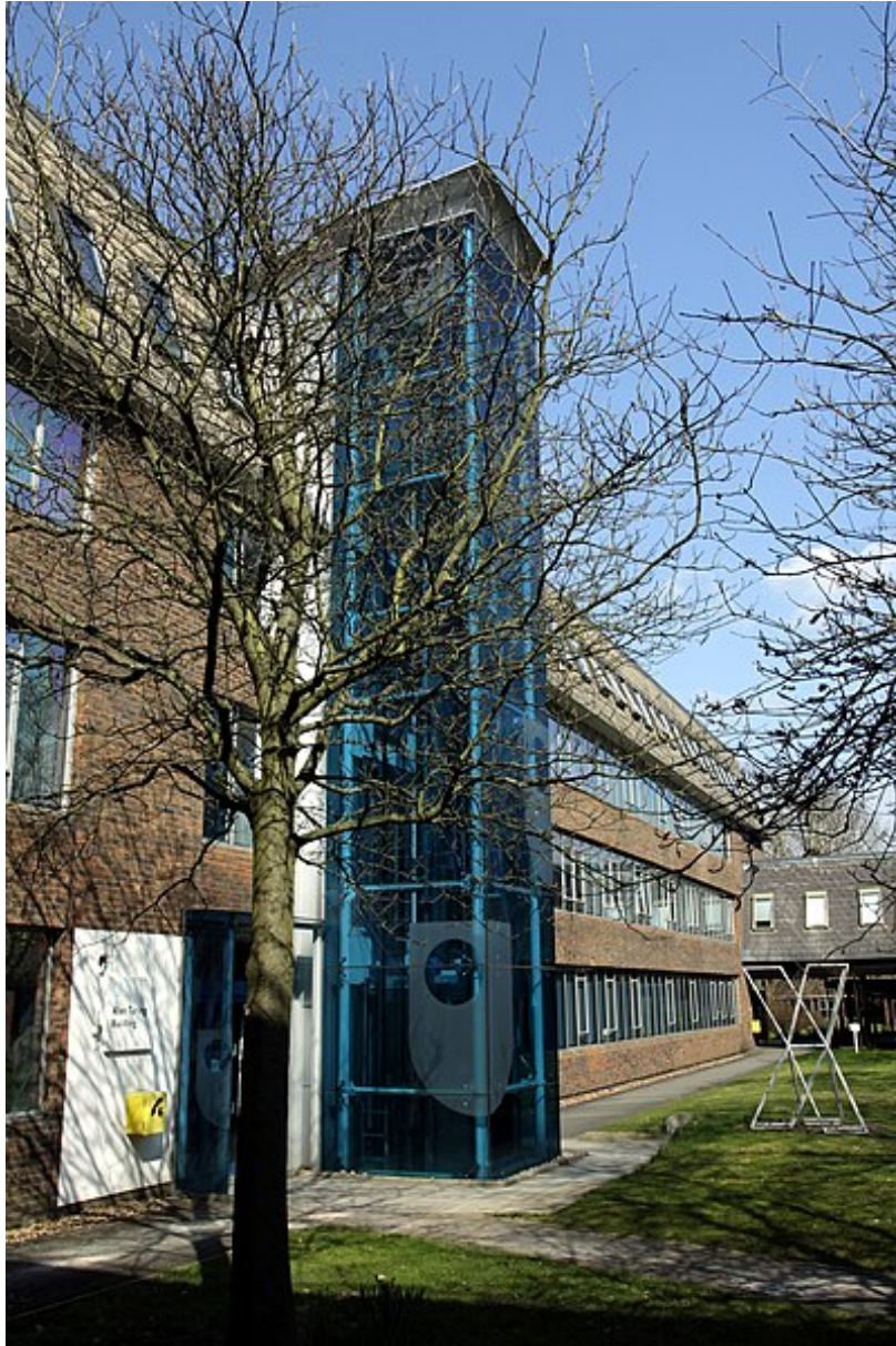
Alan Turing Building at Open University Campus in Milton Keynes, Spring 2013
